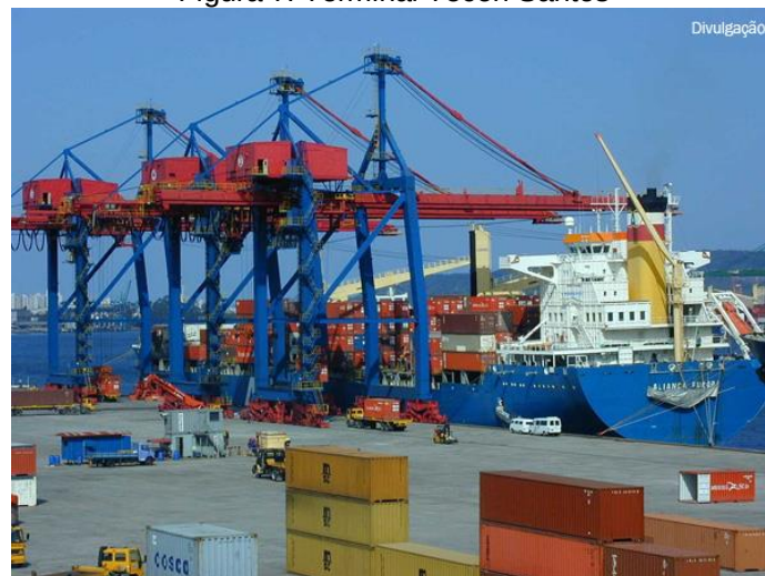
Figura 7: Terminal Tecon Santos
